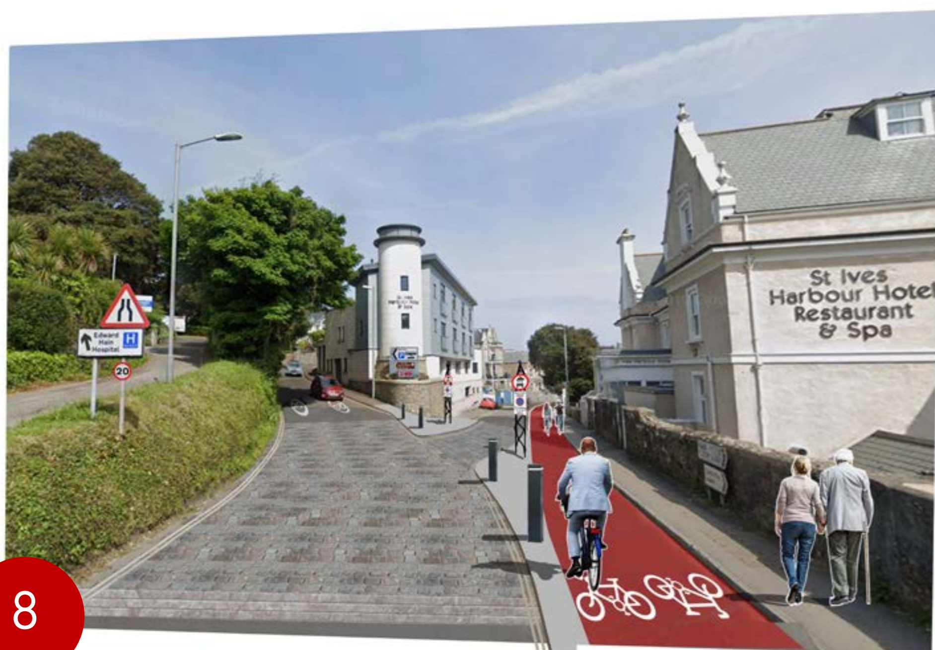
Trelyon Avenue/ The Terrace (Harbour Hotel) - 2 way cycle track and junction realigned to reinforce the vehicle restricted area in the town centre.
