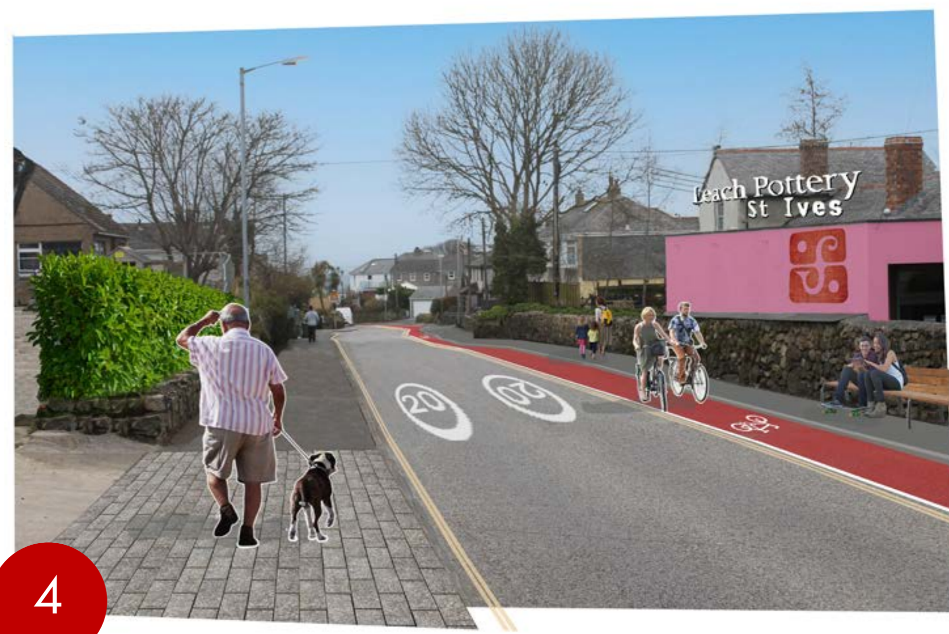
Higher Stenanck (Leach Pottery) - new footway and cycle track connects Palemon Best recreation ground with the skatepark and orchard to the rest of the town. Narrowed carriageway and slower speed limit.
